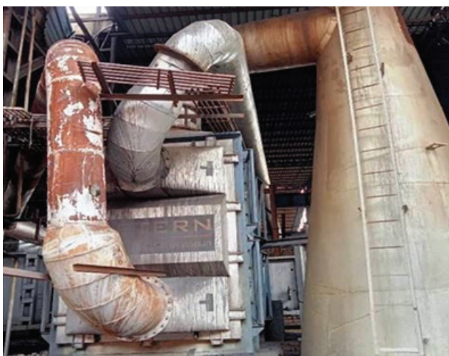
Recuperator for waste heat recovery and reuse
